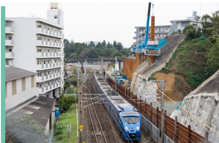
Retaining Wall Construction Work with Gyro Piler
