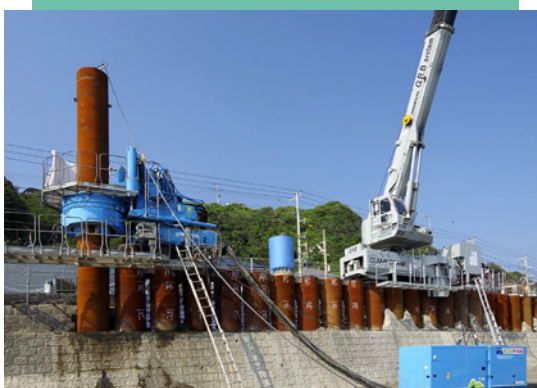
Levee Reinforcement Work with Gyro Piler
