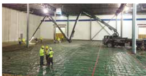
Concrete pouring at PH Inc
